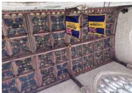
Restored panelled roof
