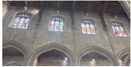
Clerestory Windows, Martyrs & Confessors of the faith
