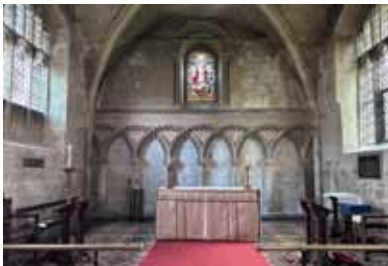
Quadripartite vault at the East end
