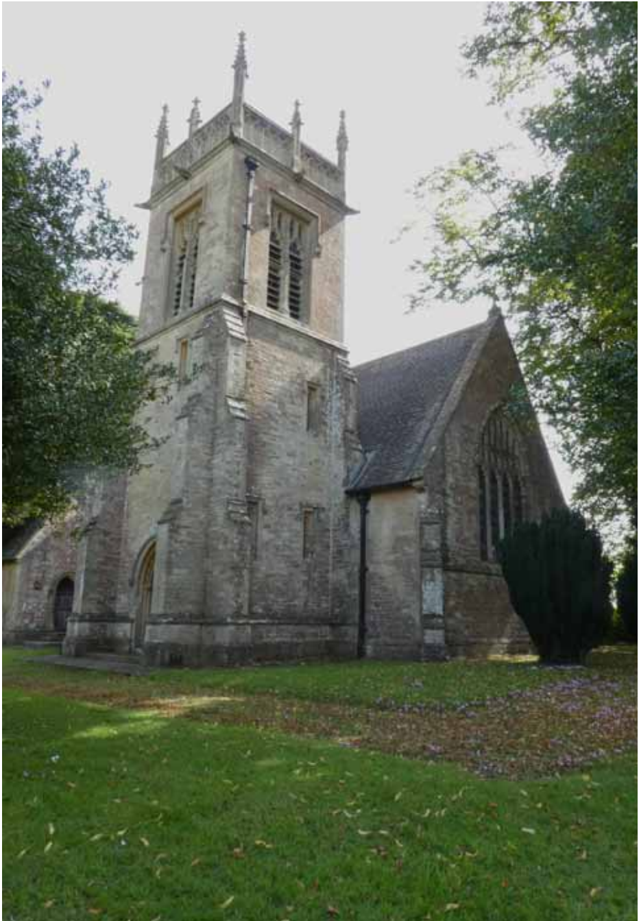
Hartham Church is a rather remarkable building, quite as large as many parish churches, built in 1862 as the private chapel for the Hartham Park Estate at Corsham. It is a Grade II listed building.
